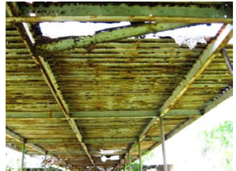
23-Apr-2010 Covered Walkways
