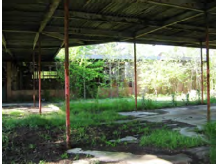
23-Apr-2010 Covered Walkways
